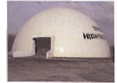
Brown County's 5,000 ton salt dome.
